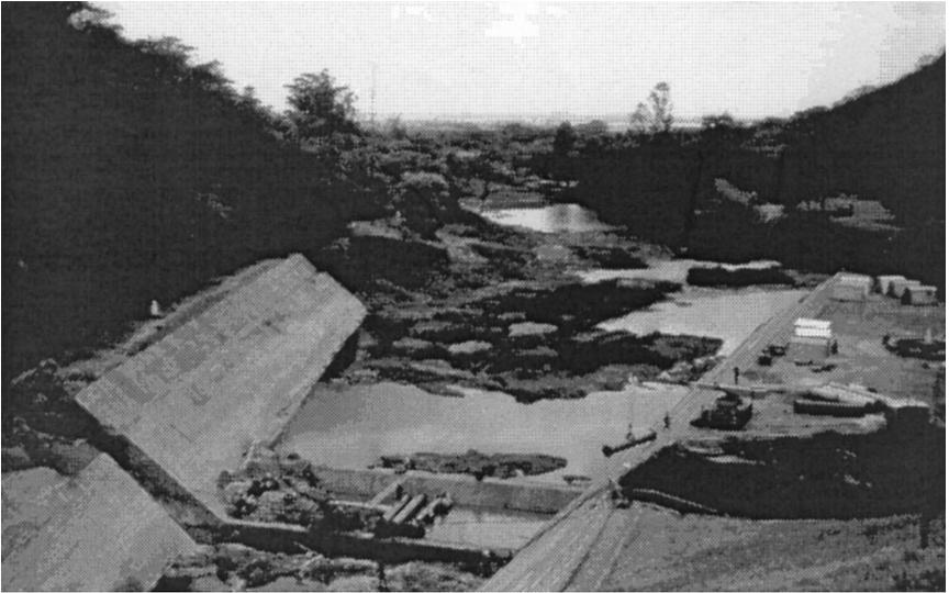
Fig. 2. The destruction of the dam in Harare's water reservoir due to water hyacinths. Photo: Nils Kautsky.
